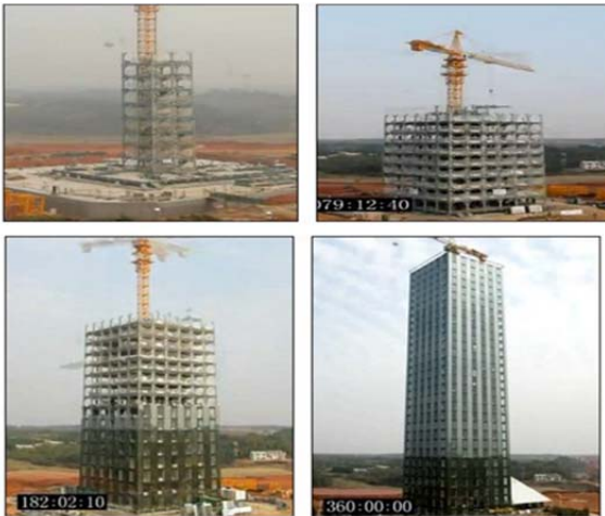
Fig.12 Overview of the rapid constructed 30 storey hotel building construction process (Sources: A Chinese Miracle 30-storey hotel in 15 days... http://thefabweb.com/16814/a-chinese-miracle-30-storey-hotel-in-15-days )
