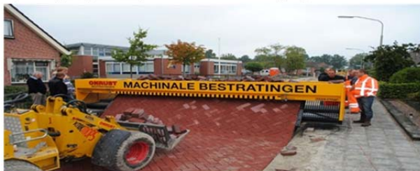
Fig. 16 Vacuum clamping machine placed the kerbstones as per alignment (source; http://www.vacuumbestrating.nl/ )
