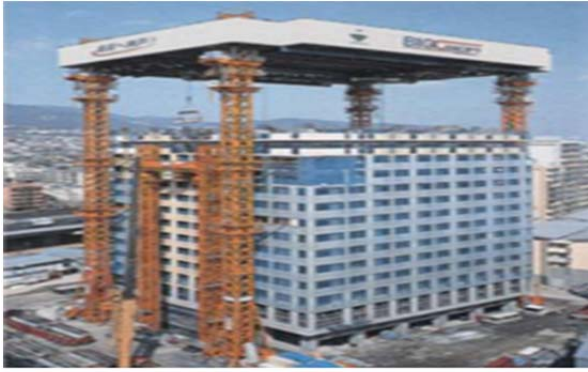
Fig 7. Overview of the BIG CANOPY automated construction factory. (Sources: www.obayashi.co.jp)
