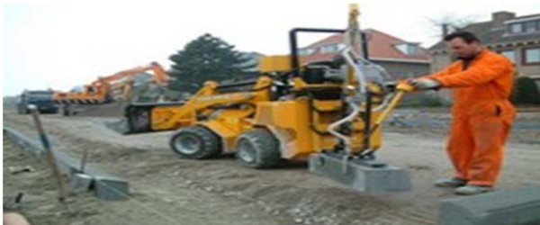
Fig. 15 Automated paving machine (source; www.google.co.in/machinale_bestratingen )
